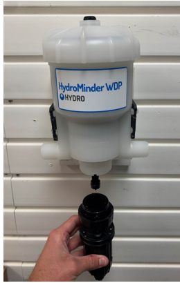
Step 1. Unscrew and remove lower end from assembly.
