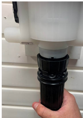
Step 8. Replace lower end assembly.
