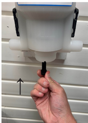
Step 7. Place shaft into the motor piston and rotate shaft 90° to lock into place. Gently pull down to ensure shaft is locked.
